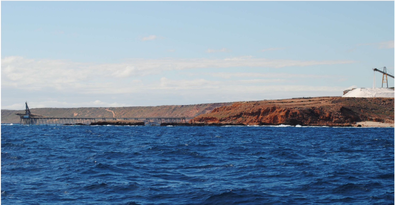
Cape Cuvier salt loading facility - mooring buoys are located other side of the jetty (R&L Newton)
