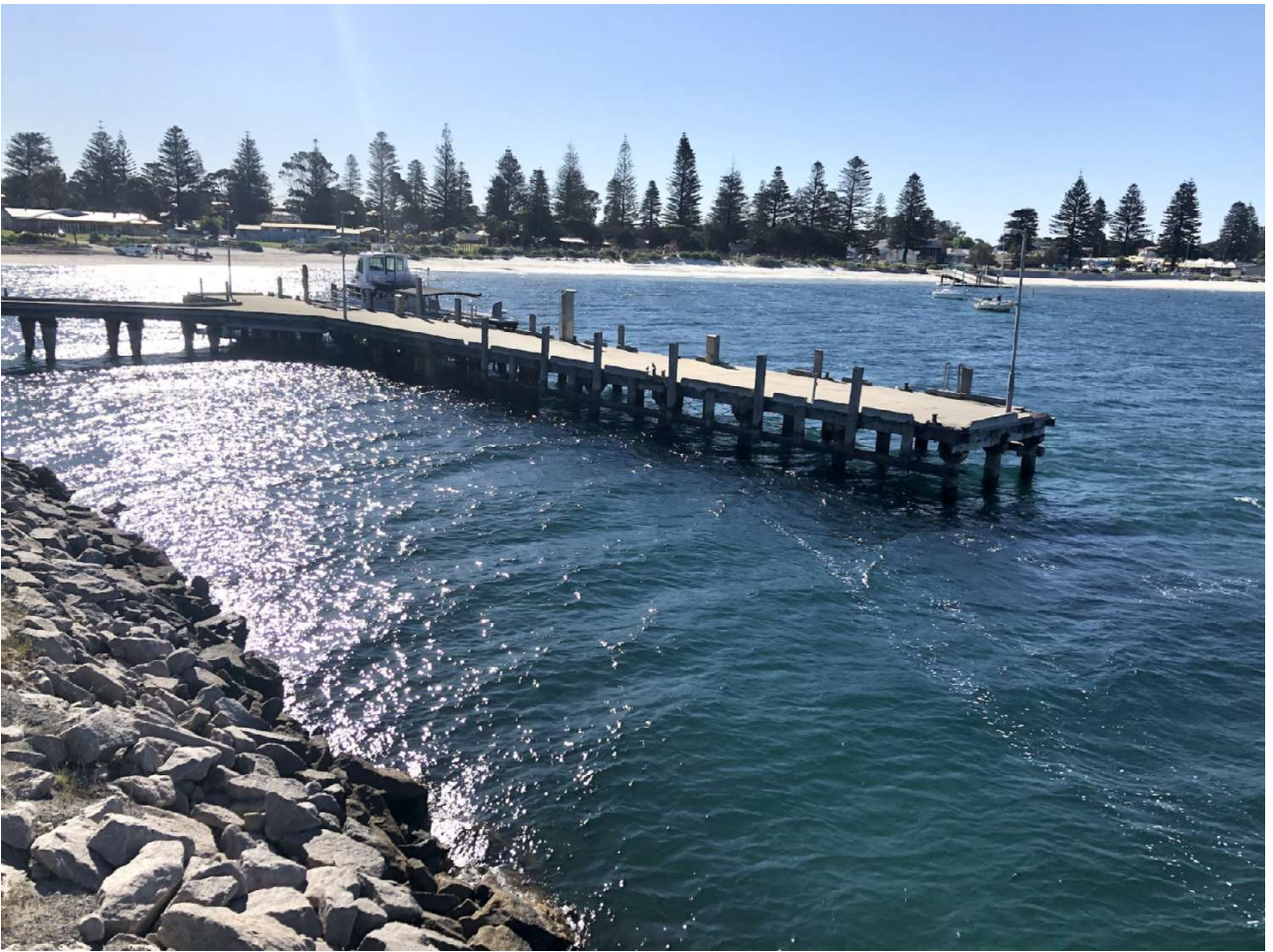
Service jetty on north side of marina (I Howlett)
